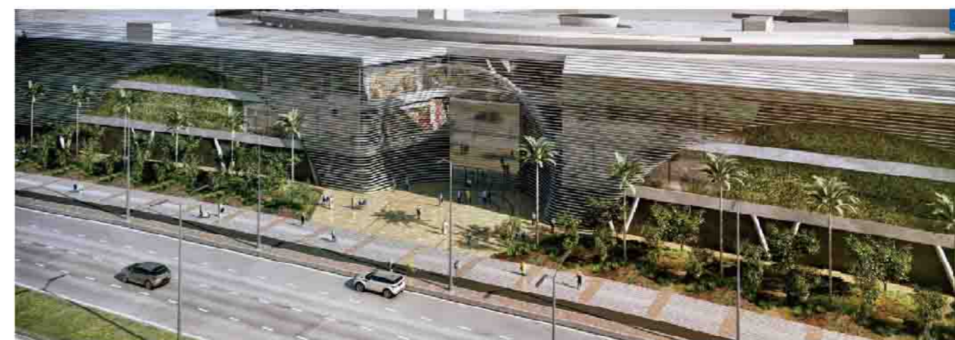
4 | Centro Comercial Parque La Colina - Colombia The Centro Comercial Parque La Colina – multiple stores is located in Bogotá. The covered area is 210.000 square meters and the construction area is 64.000 square meters. Equipment installed: 8 escalators, 5 freight elevators, 2 panoramic elevators and 2 passenger elevator.
