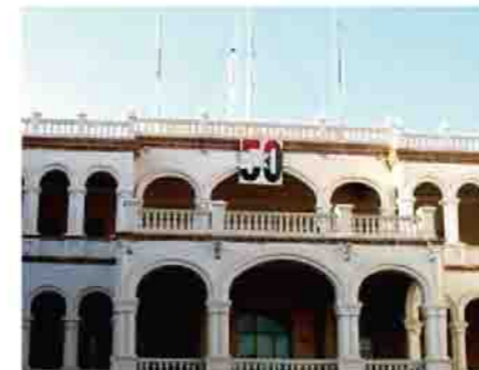
Dhaka-Government office building
